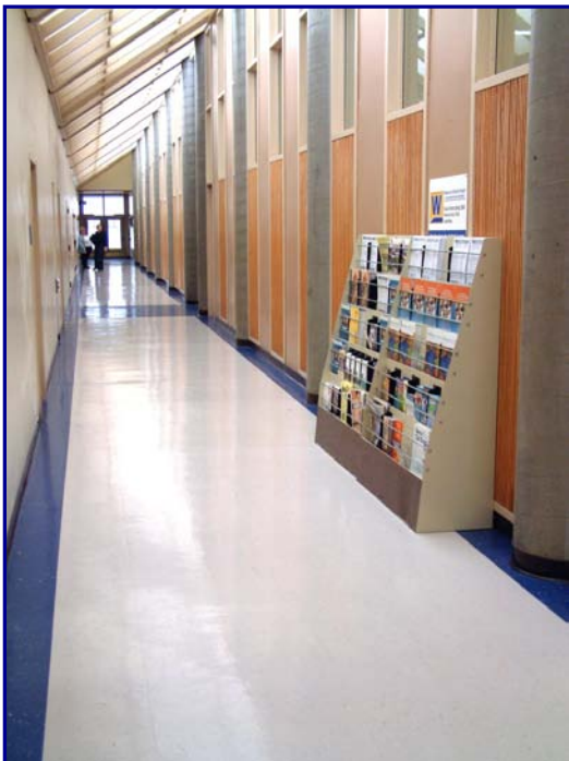
Macmillan Hall Flooring Replacement
