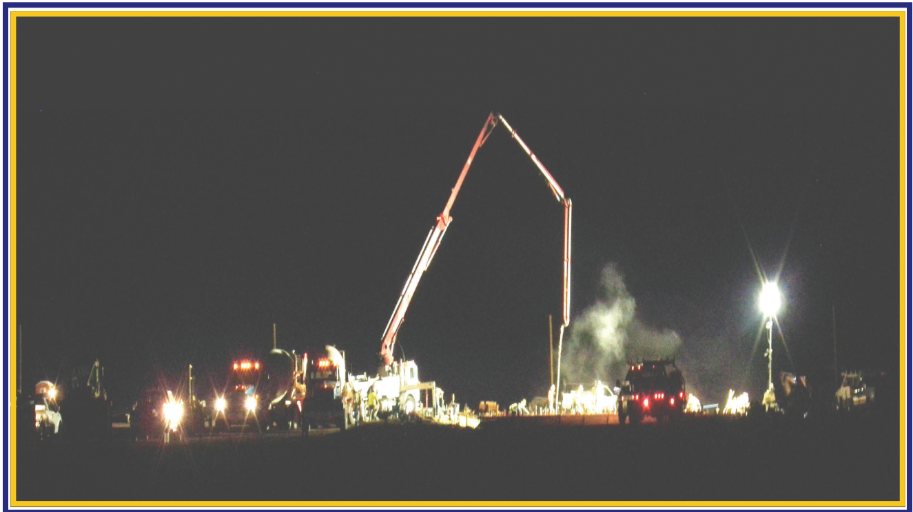
LAKE COUNTY CENTER EARLY MORNING FOUNDATION POUR
