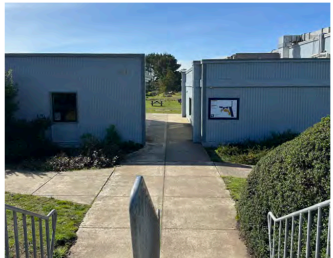
Building 100 &amp; 200 Entrance
